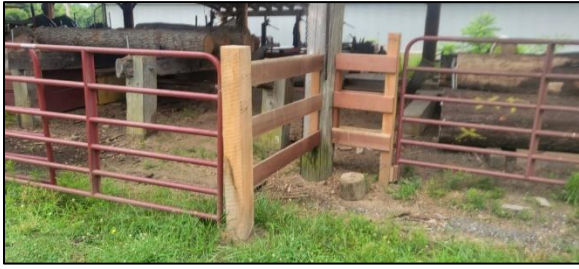
New Fence Posts and Boards
